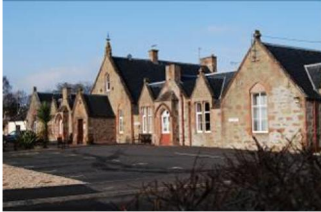
Fig 2 The Ross Memorial Hospital, Dingwall
